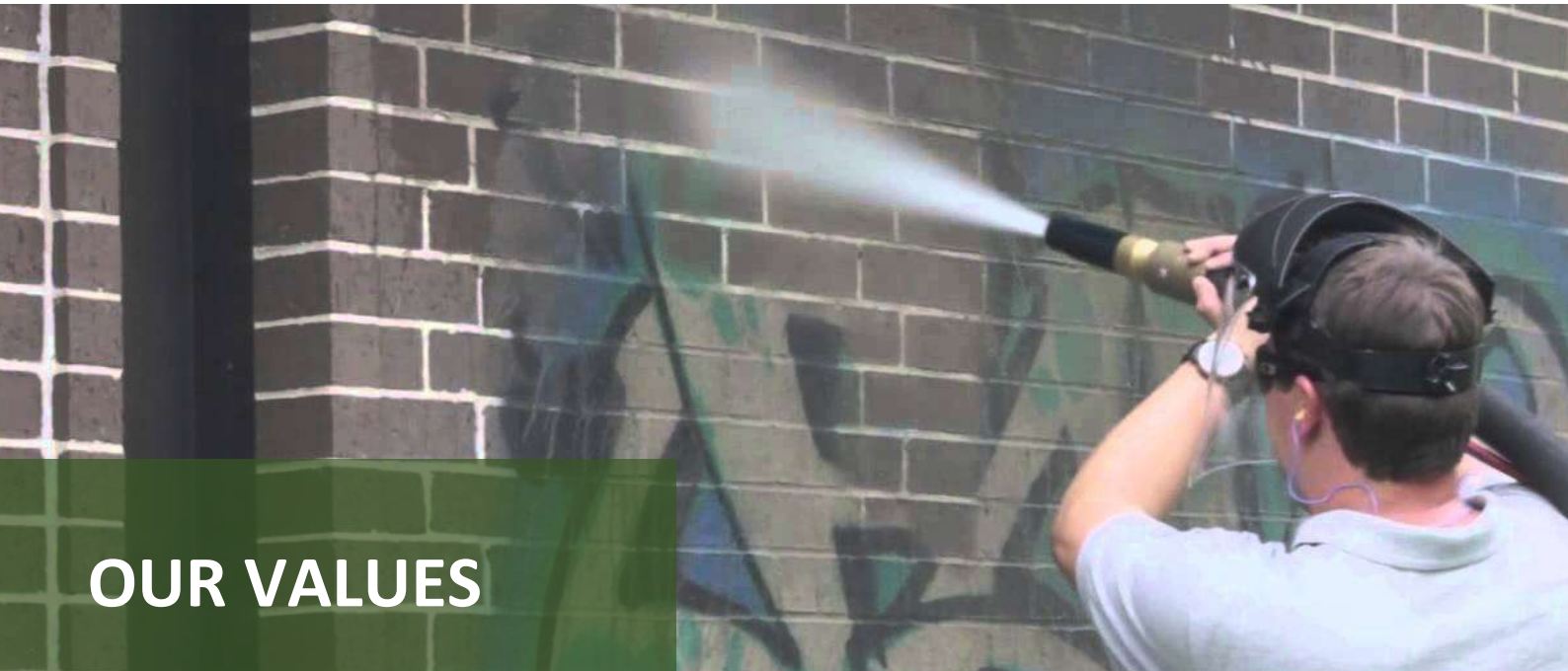
Removing graffiti from brick wall
